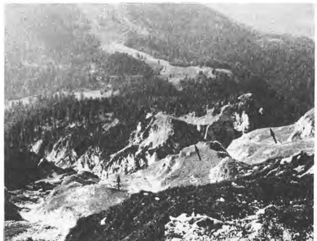
Fig.13. Toppling giant rock block at the Reißkofel (view downhill)
