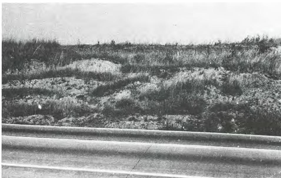
Figure 7. Shallow landslide in fissured clay, express highway Brno - Prague. The clay forms a "pocket" in crystalline rocks, thickness of the clay - 12 m.
