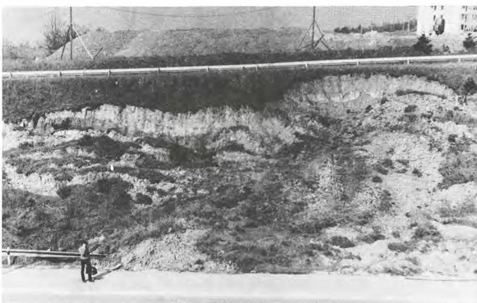
Figure 8. Landslide on the border of the loess and neogene fissured clay, highway Brno.
