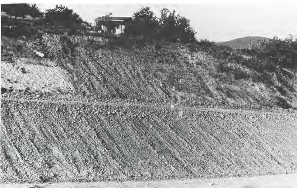
Figure 9. Stone bench at the foot of the slope as the stabilization of the landslide in fissured clays, reconstruction of the tramway line, Brno.
