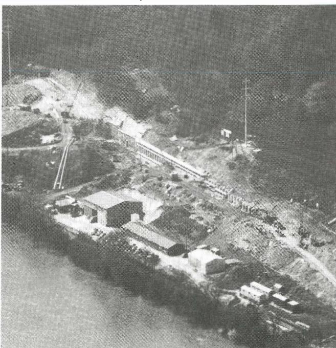
Fig. 1 North portal of the Born tunnel with anchored pile wall and ground freezing (photo SBB)
